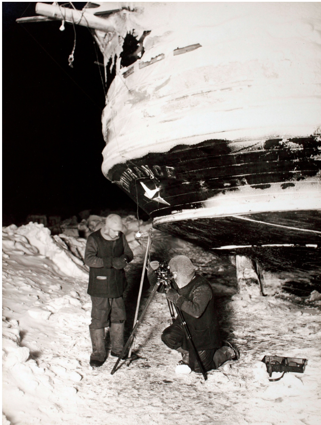
Figure 1. Captain Frank Worsley (left) and Reginald James taking sights from the sea ice by the stern of Endurance . Worsley cradles a chronometer or stopwatch and James uses the theodolite to measure the altitude of a star. Scott Polar Research Institute, University of Cambridge, with permission. Photograph by Frank Hurley, 1915. All rights reserved.
